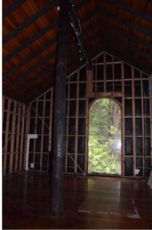
Figure 13: The Māori Hall, with wall linings removed. Note central supporting pou, and arched window representing the 'eye of Rua Kenana'.
